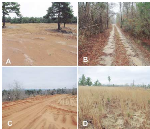
Figure 2. Photographs illustrating typical heavy-machinery training areas (A), trails (B), unpaved roads cover (C), and nonforested land (D) at the Fort Benning Military Installation, Georgia. Note the unstable, vegetation-poor soils in A and C, the poorly defined road cover in C, and the exposed (unvegetated) soil in D.
