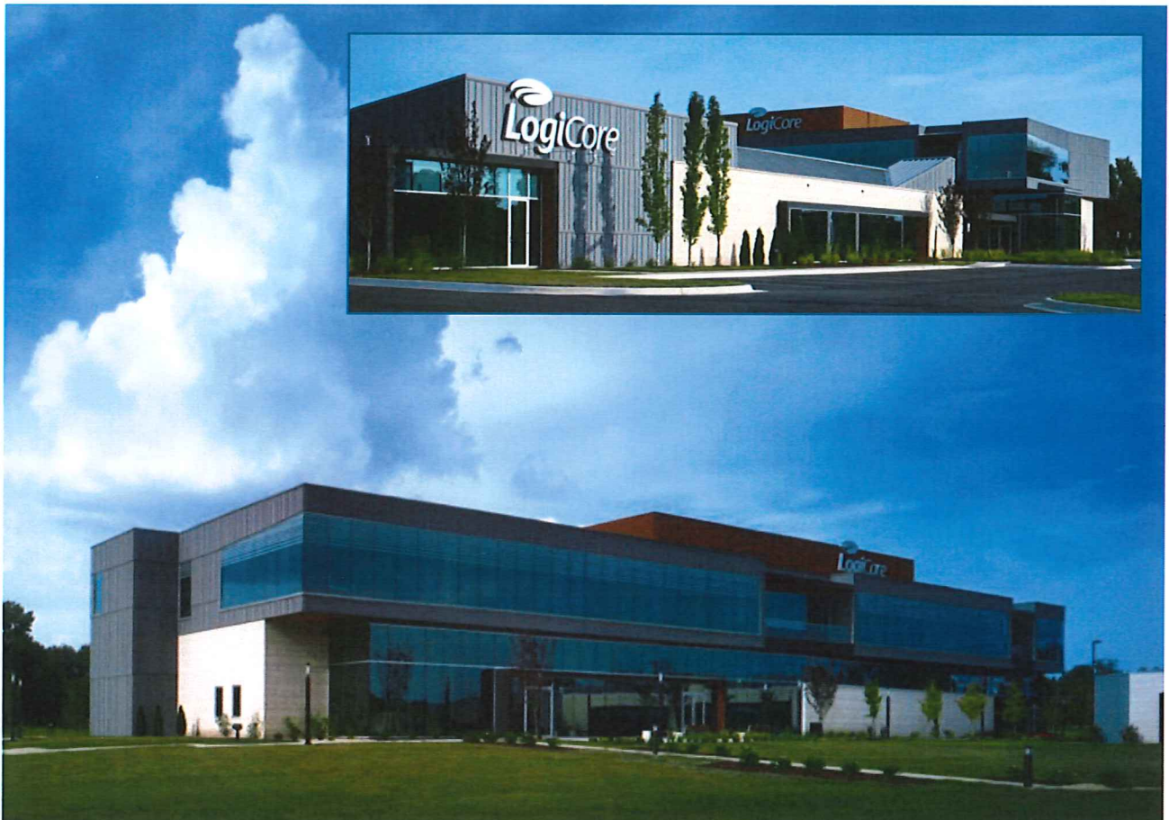
Figure 2. Ground views of LogiCore buildings.
