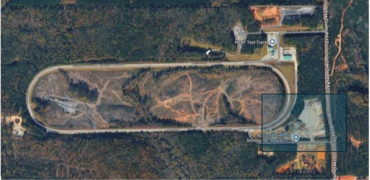
Stormwater Testing Facility
